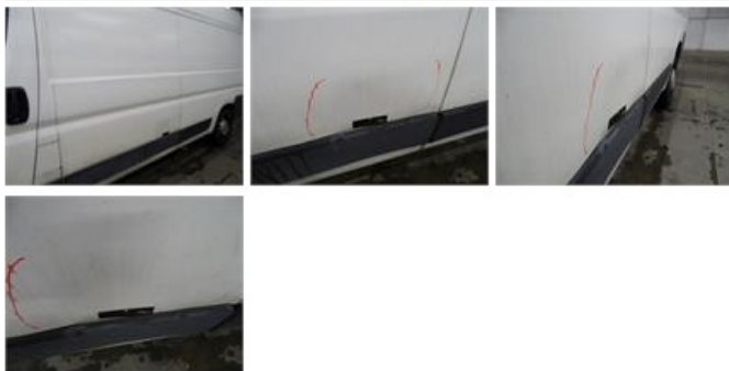
Trunk door panel L, Broken, E - Replace
